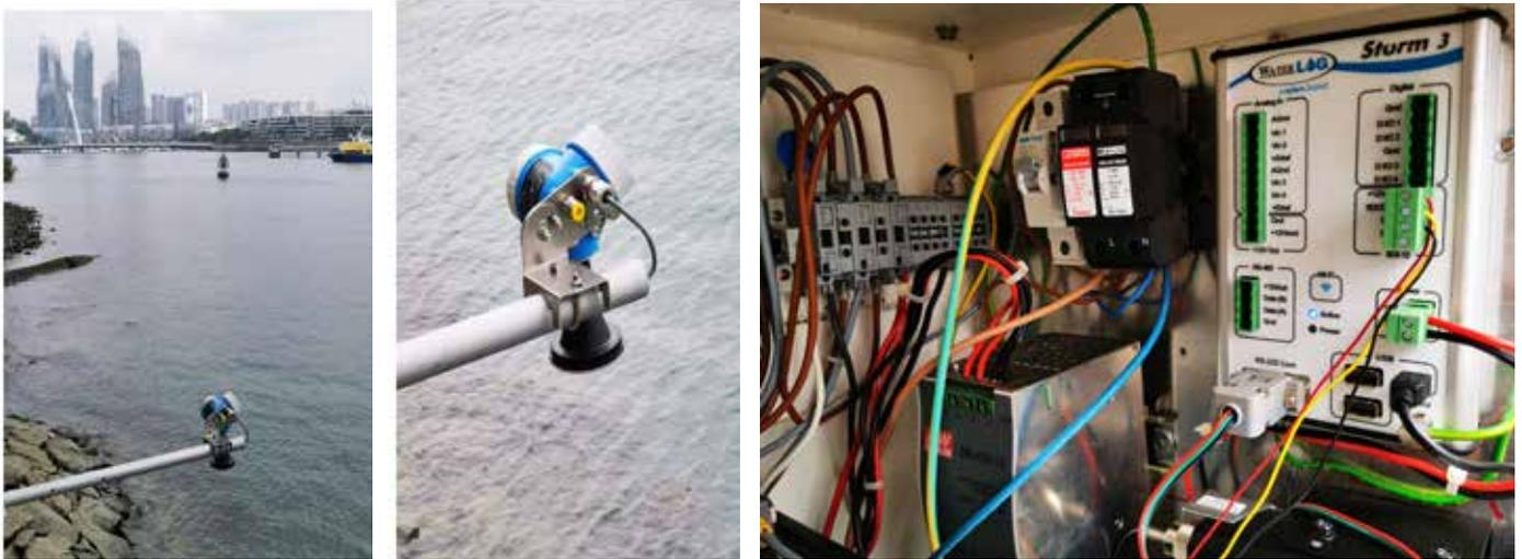
SINGAPORE: Nile Radar level sensors installed upstream and downstream of the Marina Barrage measuring real time tide and reservoir levels.
