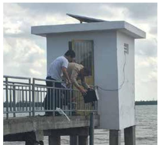
**Fig. 2.** Installation of Nile Radar Water Level Sensor
